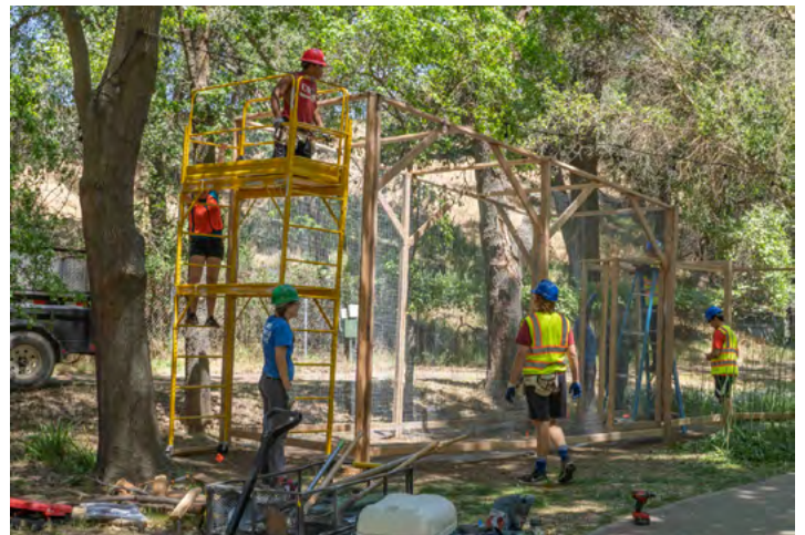
Students begin work on the flight cage structure.
