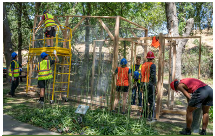
The cage frame and screens take shape.
