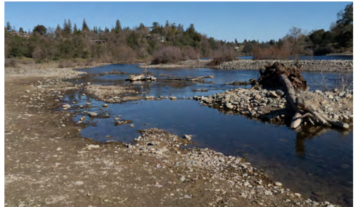
A rearing alcove was created adjacent to the river to protect juvenile fish.
