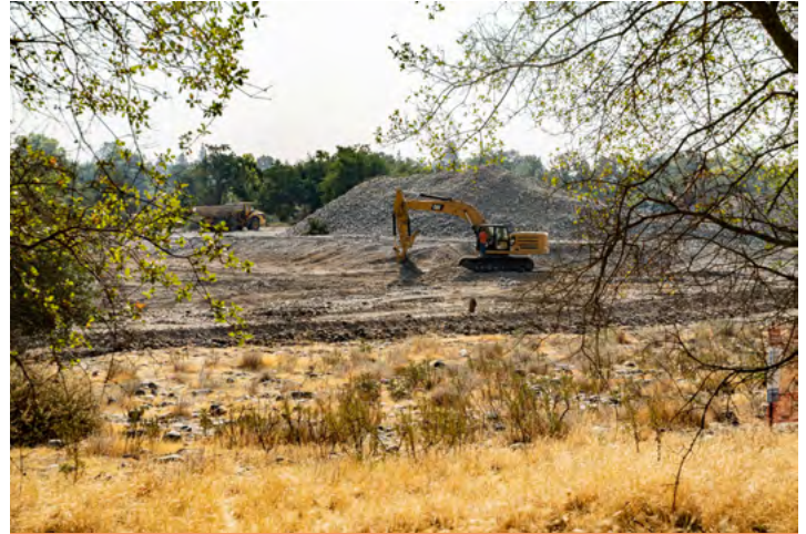
In late summer 2021 heavy machinery was brought in to move rocks and soil to create salmonid habitat.
