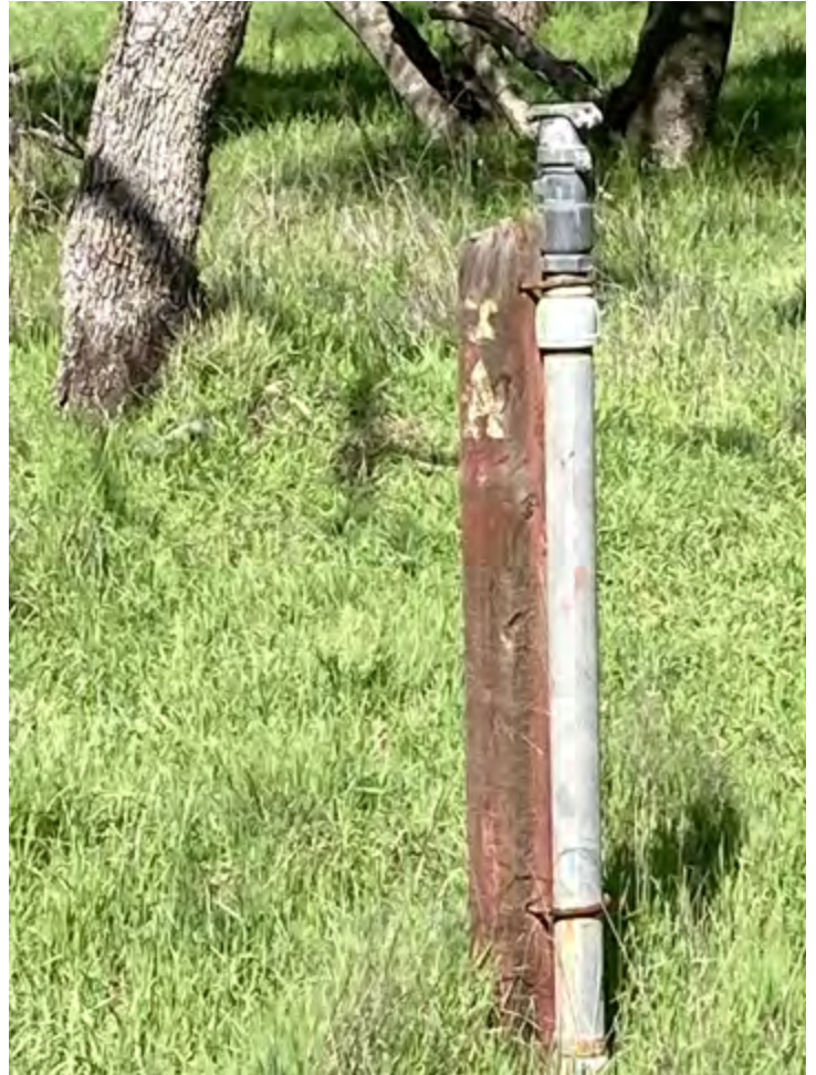
A standpipe that can be accessed to shoot water onto a fire in the NSA. Photo © Melanie Loo.
